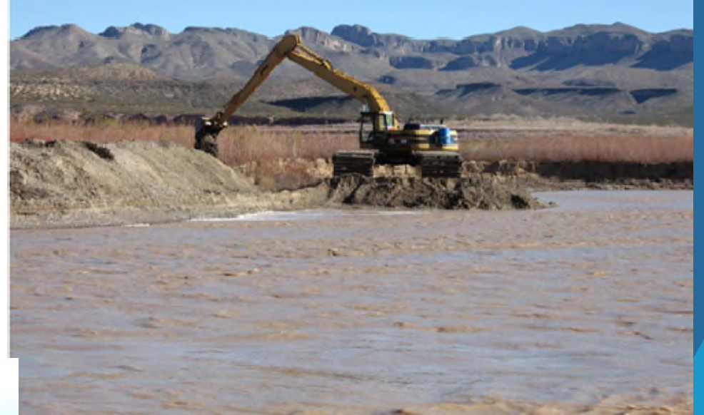
Amphibious caterpillar terracing the bankline
