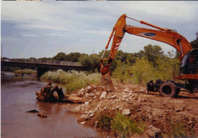
Figure 14. Installation of cottonwood snag structures. Top Left: Snag is uprooted and transported to stream bank. Top Right: Snag placed in excavated trench with rootwad streamside. Bottom Left: Trench is re-filled with soil and rock. Bottom Right : Banks are re-sloped and rock armor placed. Site is ready for revegetation.
