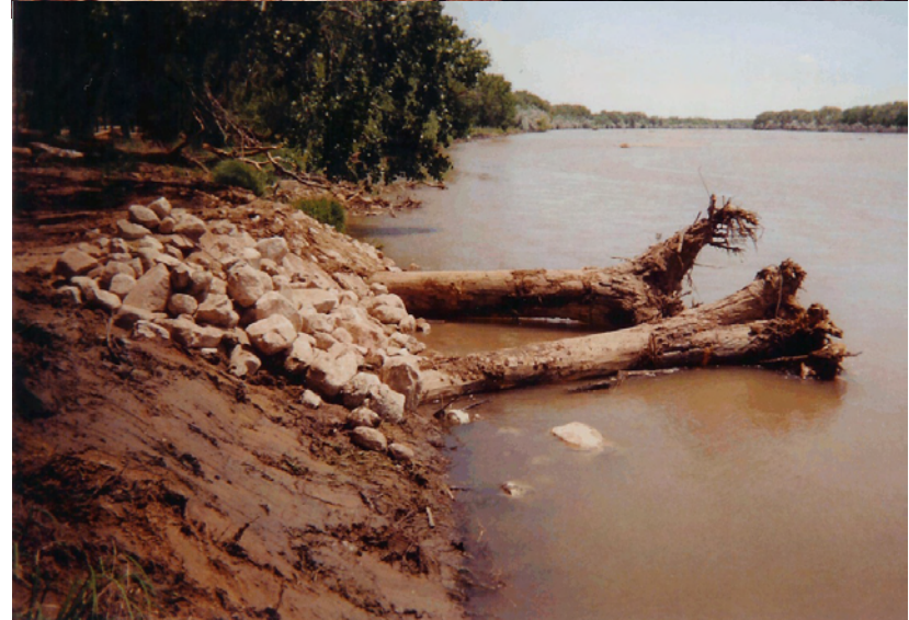
Figure 14. Installation of cottonwood snag structures. Top Left: Snag is uprooted and transported to stream bank. Top Right: Snag placed in excavated trench with rootwad streamside. Bottom Left: Trench is re-filled with soil and rock. Bottom Right : Banks are re-sloped and rock armor placed. Site is ready for revegetation.
