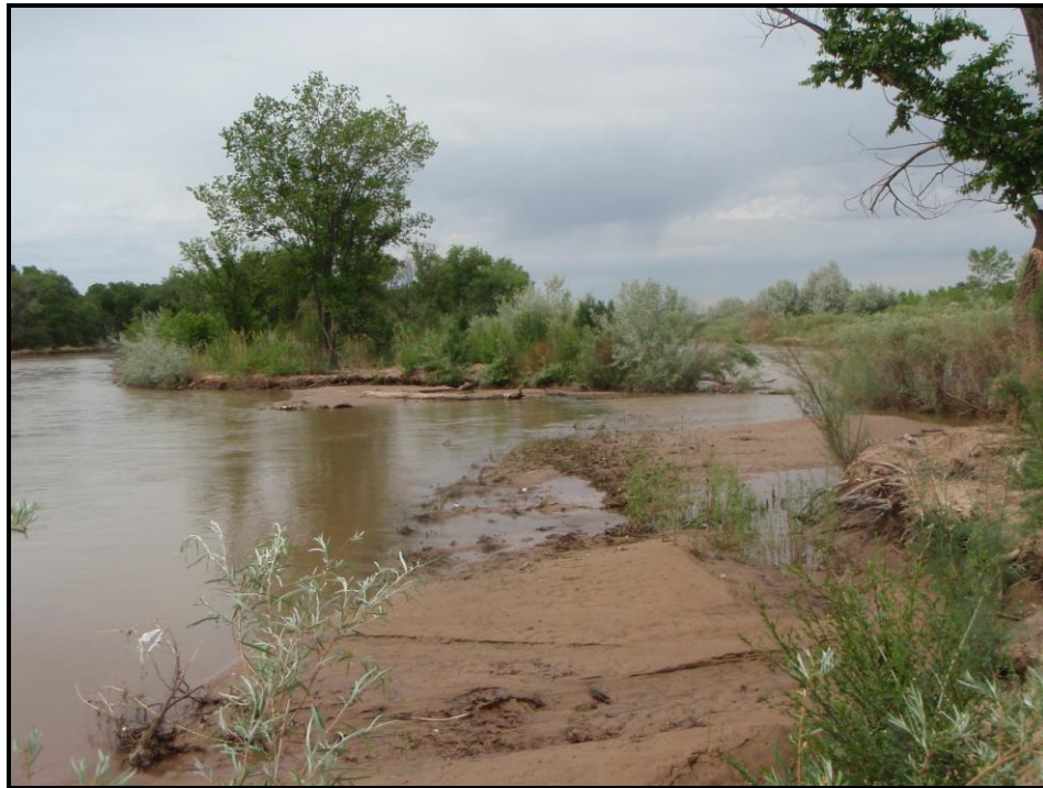
Figure 19. The effect of erosion at Scallop #2 at the RBS site. This scallop is now connected to the constructed channel at high flows (south orientation).
