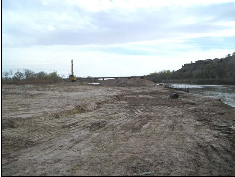
Figure 2. Excavator moving spoil into embayment at I-40-2i.
