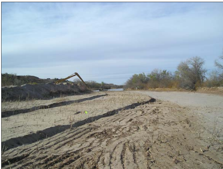
Figure 3. Excavator creating terraces at I-40-2i.
