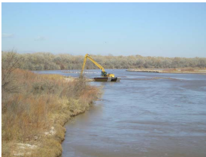
Figure 13. NDC-5i creation of silt curtain and embayment.
