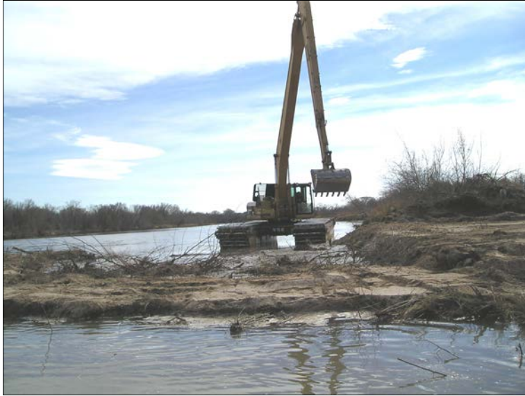
Figure 5. Excavator moving spoil and excess vegetation to build silt curtain at SDC-4i.
