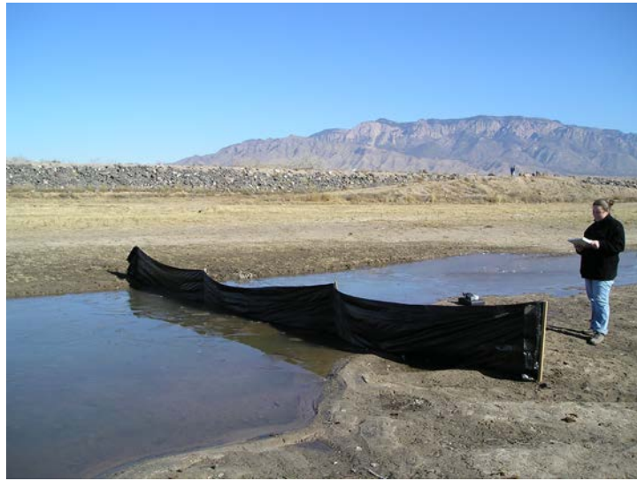
Figure 13. Silt fencing used while crossing the North Floodway Channel.
