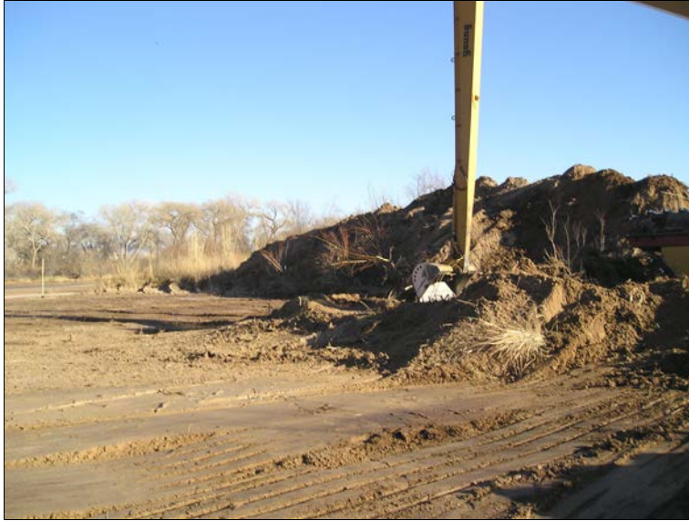
Figure 2. Excavator moving spoil and creating contours at SDC-2i.
