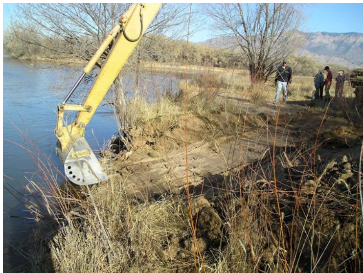
Figure 14. Construction of a ramp to access the Rio Grande from Sandia lands.
