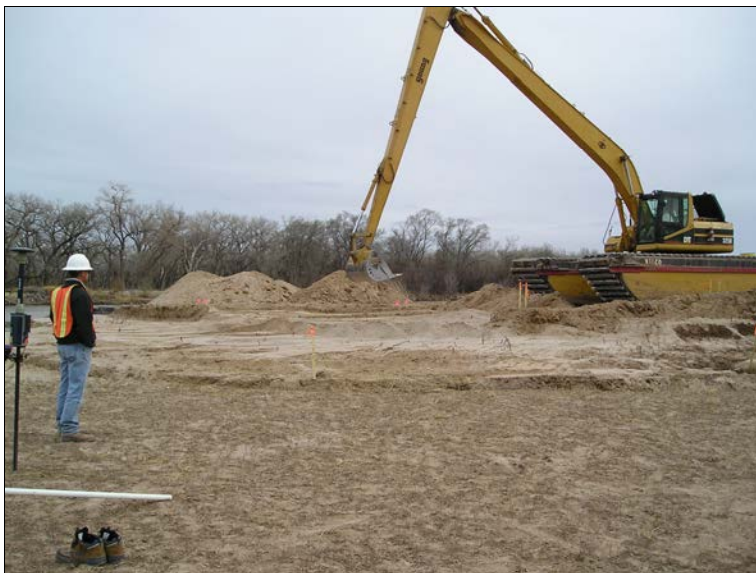
Figure 6. Excavator moving spoil to create terraces at SDC-4i.
