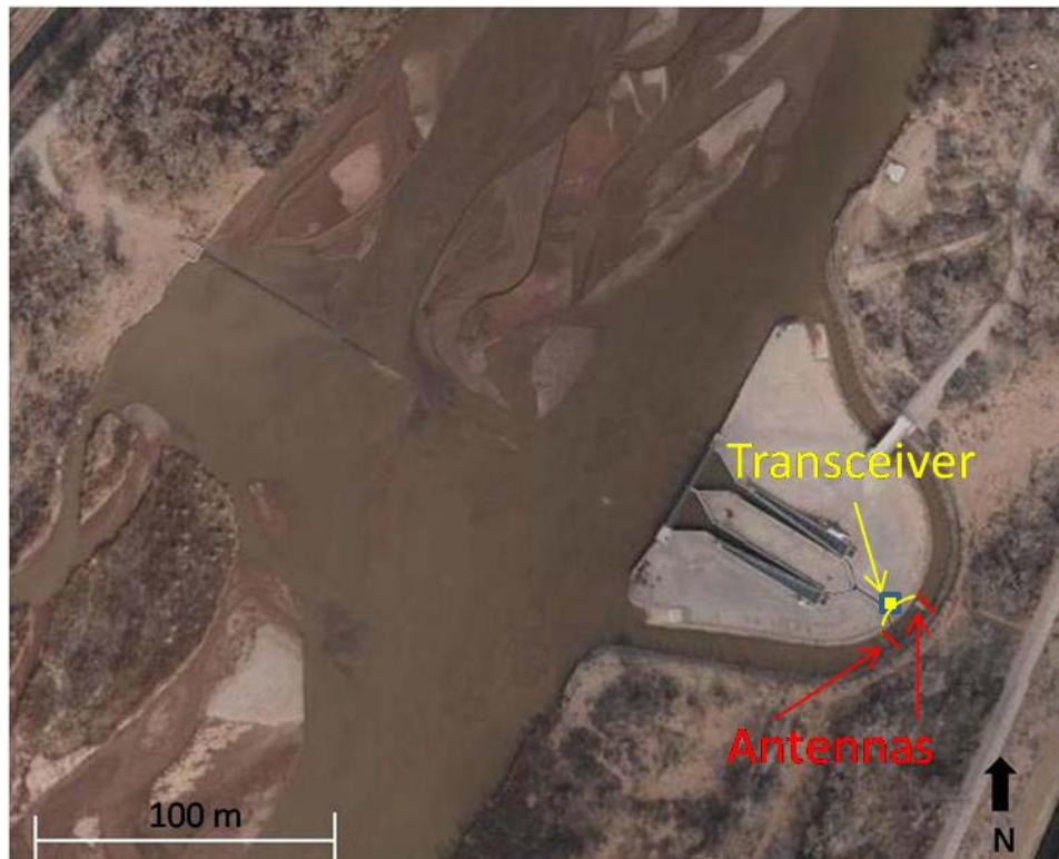
Figure 2-Aerial view of the Rio Grande drinking water diversion and fish bypass channel in Albuquerque, New Mexico.
