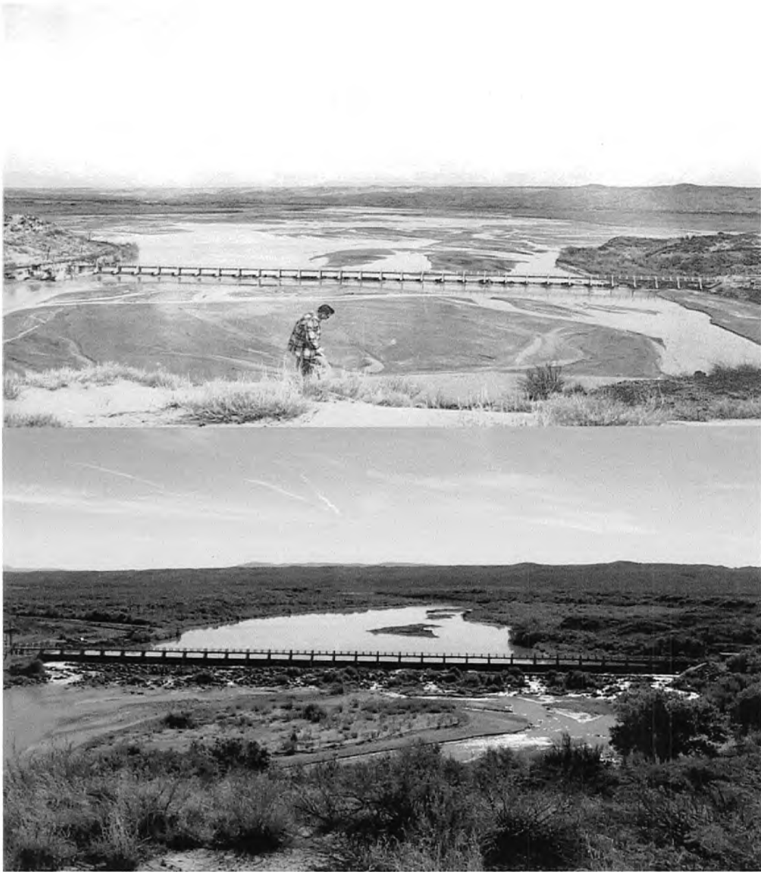
Figure 2: View of San Acacia dam 1952 and 2002 that shows how strongly the channel has been narrowed in last 50 years.
