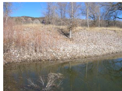
Spoil-bank levees line the east-side river channel along the Velarde Sub-Reach of the Rio Grande.
