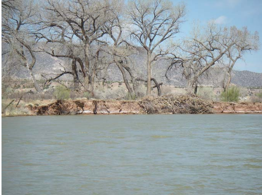
Photo: April 2008. Flow is about 1,800 cfs.
