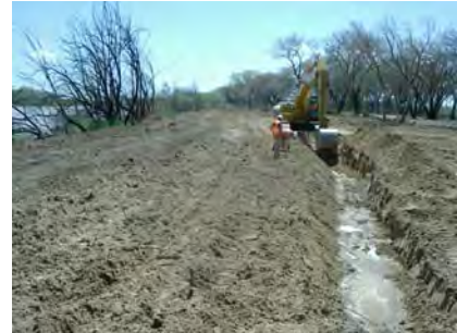
Willow swale construction near Albuquerque. (Photo Credit: Parametrix)
