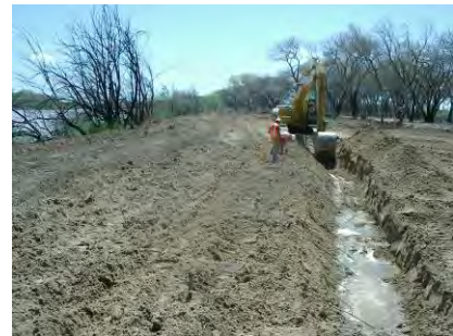
Swale construction in the Albuquerque bosque in 2005. (Photo Credit: Parametrix).
