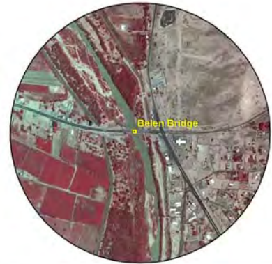
Example of constricted channel segment immediately upstream and downstream of the Belen Bridge. Areas like this are excluded from bar destabilization and lowering treatments to avoid negative impacts to the bridges.
