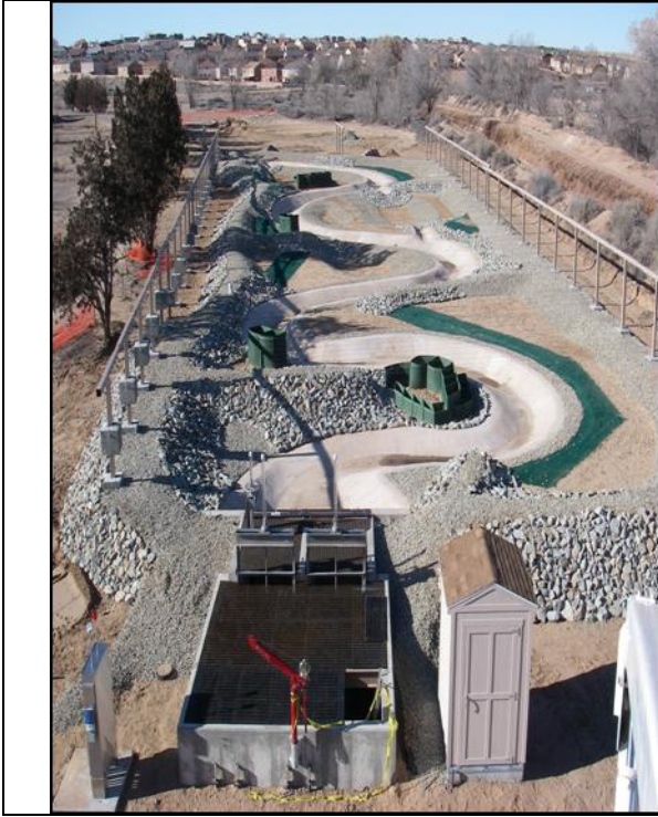
Construction of naturalized habitat at the Los Lunas silver minnow refugium.
