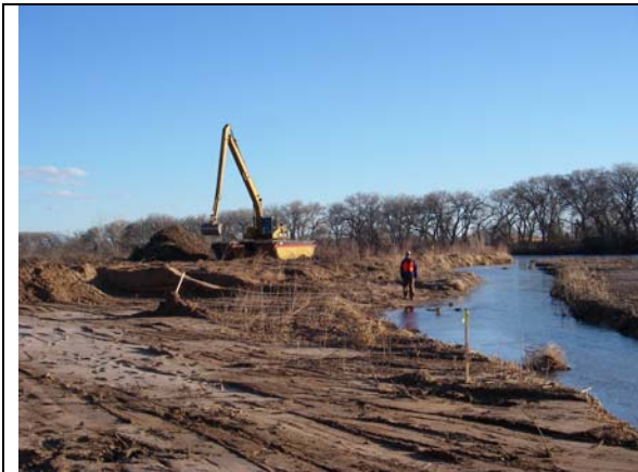
Figure 3.6.1.1. Island modification in the South Diversion Channel subreach. (Photo provided by Anders Lundahl, Interstate Stream Commission and shown is Sara Beck, SWCA)
