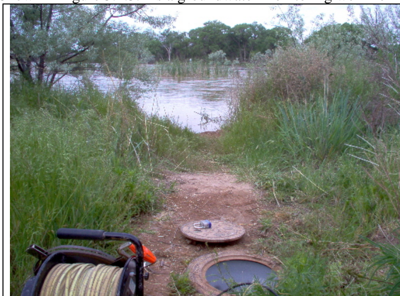
Figure 3.1.3.1. USGS Groundwater monitoring well in the riparian area of the Middle Rio Grande, Albuquerque reach. (Photo provided by USGS)
