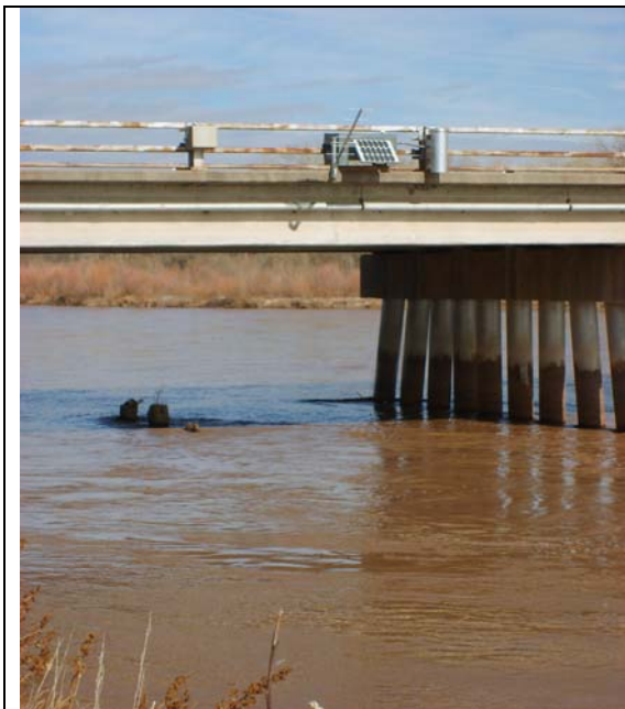
Figure 3.1.2.1. Gage apparatus located on the Highway 346 Bridge. The equipment is: A Design Analysis H-522 high-baud DCP housed in a steel Knaack box mounted on the downstream side of guardrail. A solar panel charges the battery that powers the gage. The DCP is linked to a DA H-360 radar transmitter/receiver stage sensing device. A wire-weight gage (WWG) located on the bridge guardrail near the radar unit is used as reference (Photo provided by George Sieber, USGS)
