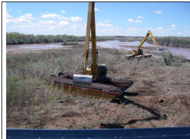
Figure 3.6.1.3. Island modification in the Paseo Del Norte subreach. The features shown are designed to inundate at river flows of 2,500 cfs or greater. The inundated shelf provides habitat to support various life stages of the silvery minnow. A shelf, approximately 8 to 10 wide, was also excavated on the northeastern bank of the island to provide additional habitat for silvery minnows at lower river flows. (Photo provided by Anders Lundahl, Interstate Stream Commission)
