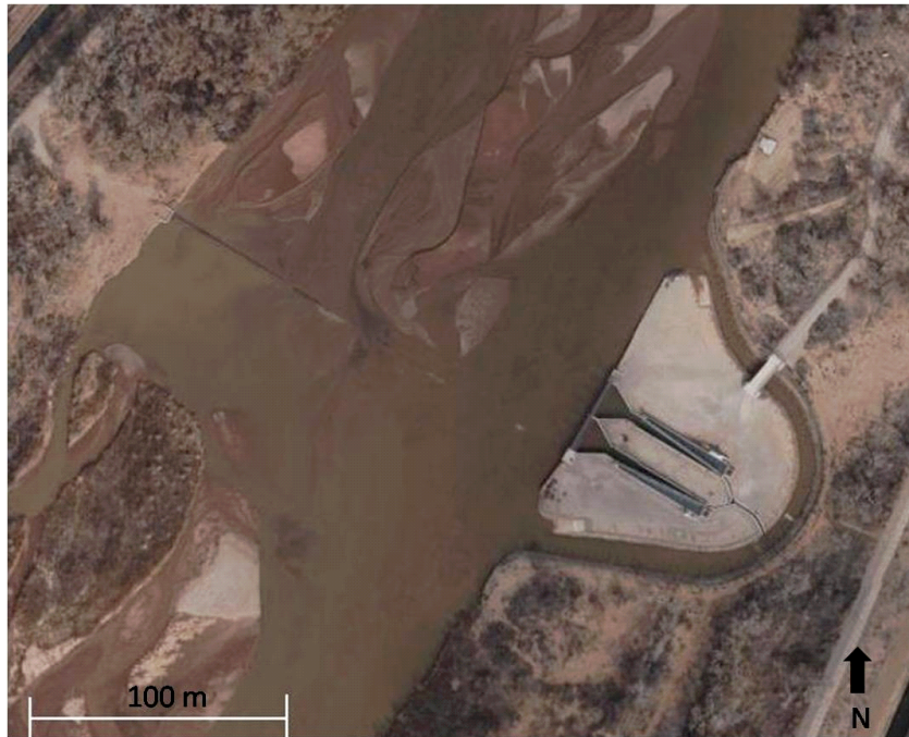
Figure 8. Alameda diversion dam and fish passage structure (Remshardt and Archdeacon 2010).
