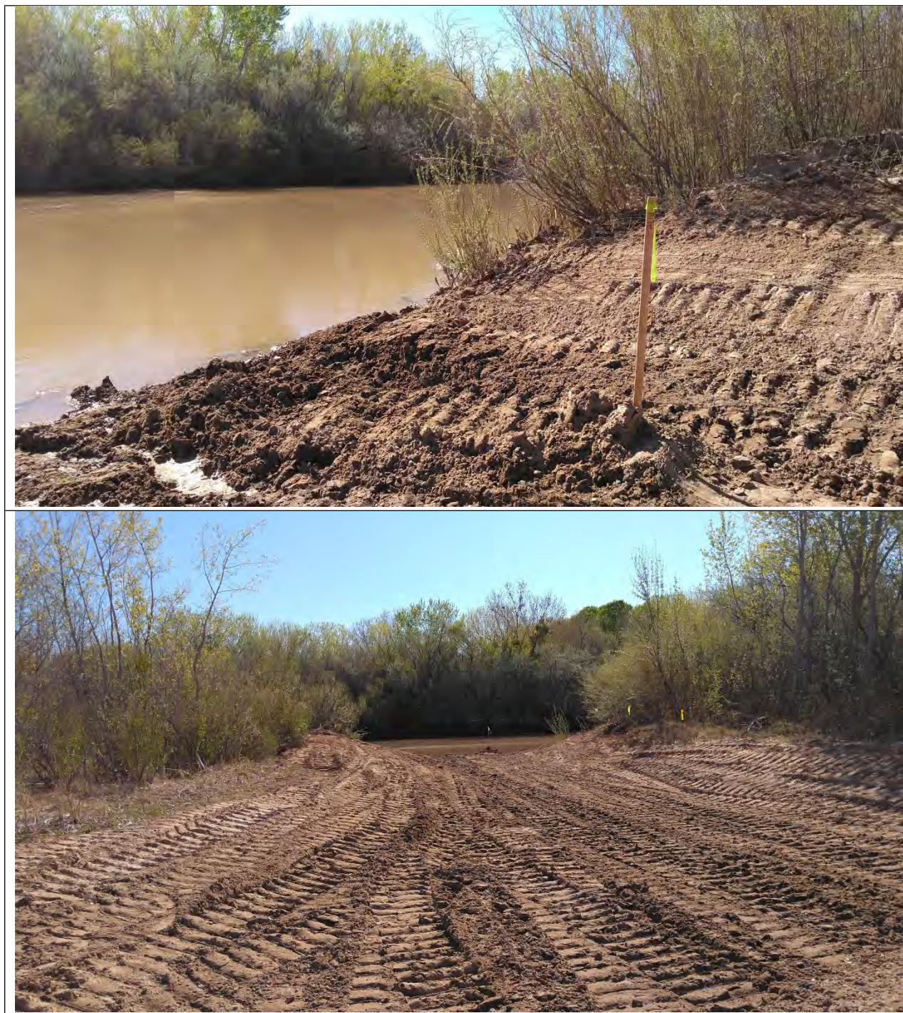
Figure 5. Representative photos of sediment removal within channel maintenance zones. These photographs were taken immediately after sediment removal at RM 100.5
