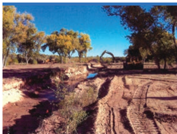
Construction on Sandia Side Channel during Oct 2009.
