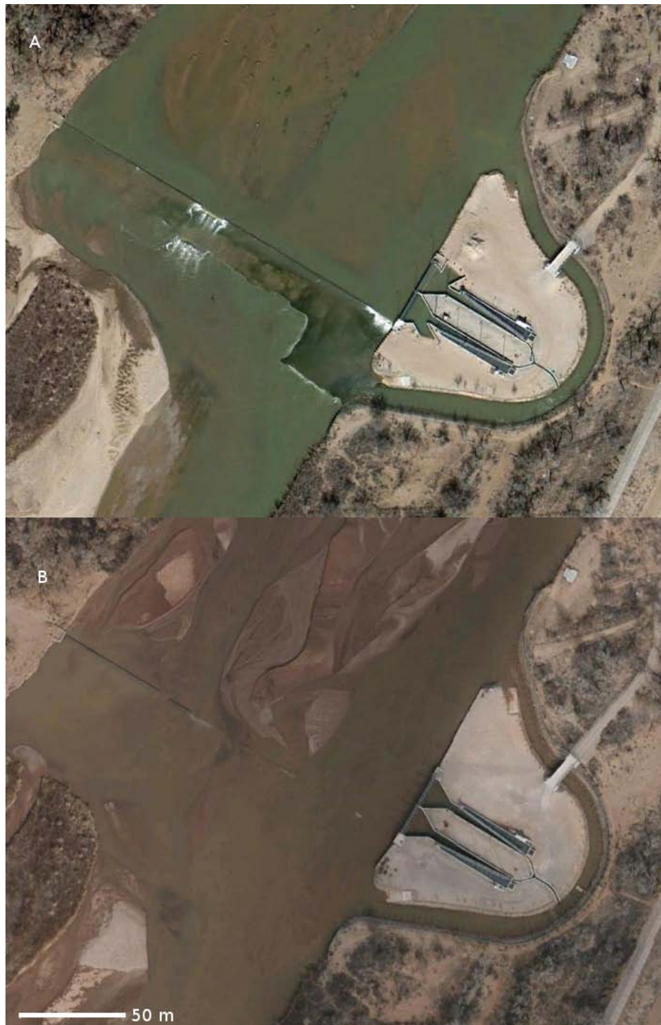
Figure 2-Fish passage structure on the Rio Grande, Albuquerque, New Mexico. A) Shows the scour pool that formed below the passage, which was filled with concrete rip-rap on 26 May 2011. B) shows the passage after completion.
