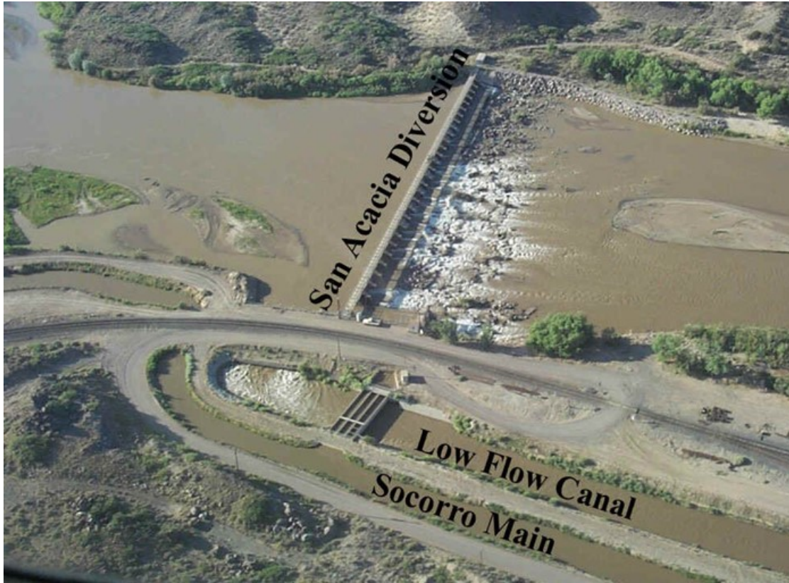
Figure 2. San Acacia diversion dam and diversion headworks. Photograph by Paul Tashjian accessed from http://www.fws.gov/southwest/bhg/images/san1.htm , November 2007
