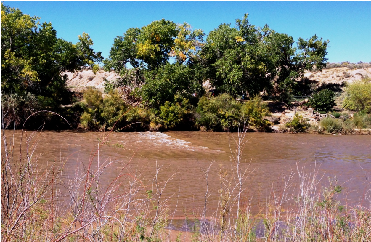
The Rio Grande flowing over the Corrales Siphon.
