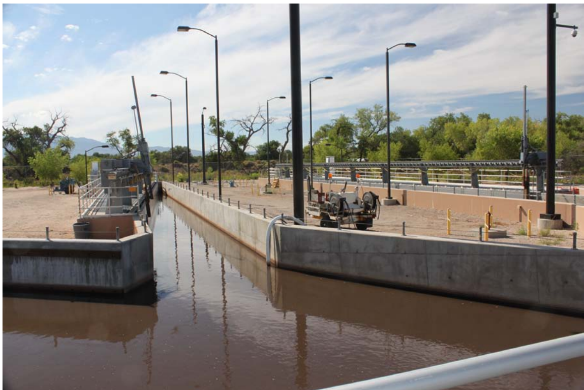
2. Looking southeast to the facility structures.
