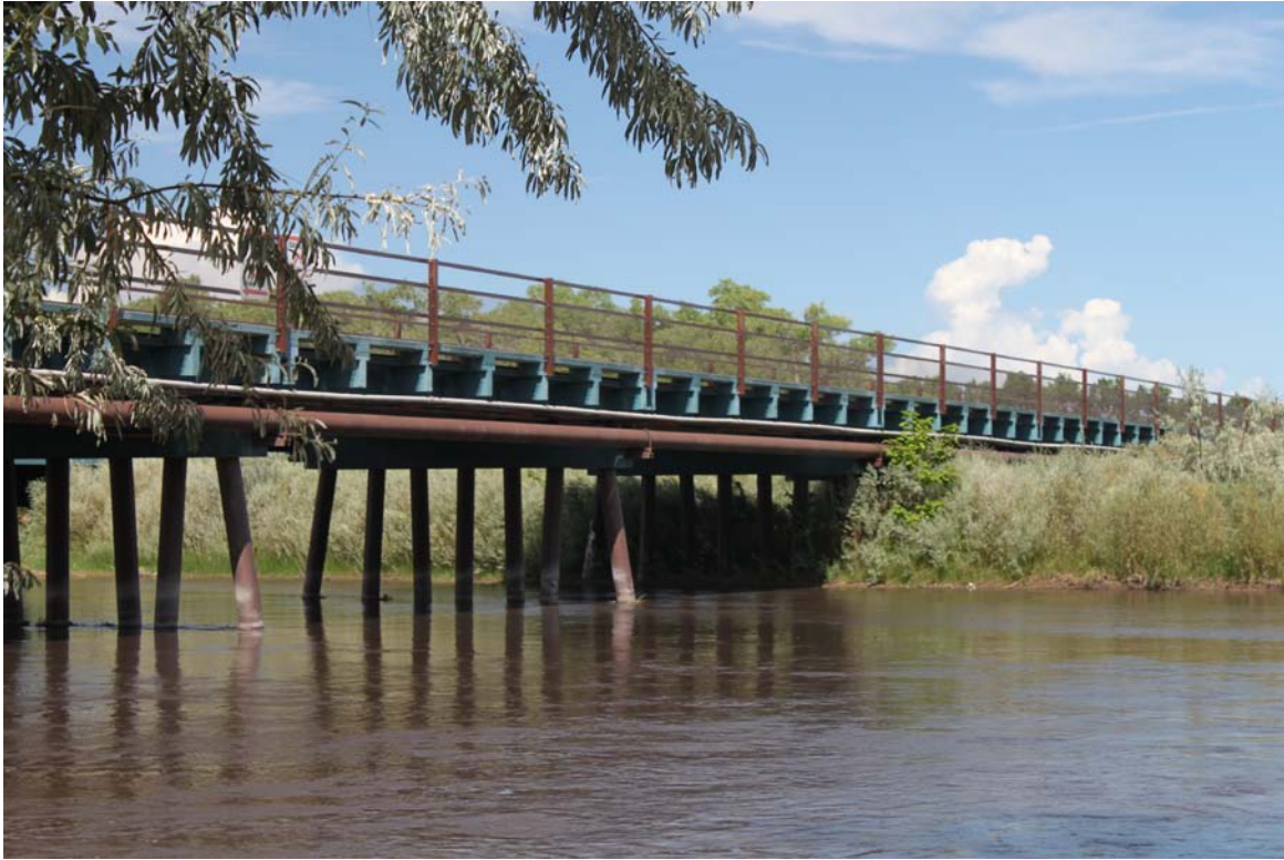
5. Looking south - Old Alameda Bridge
