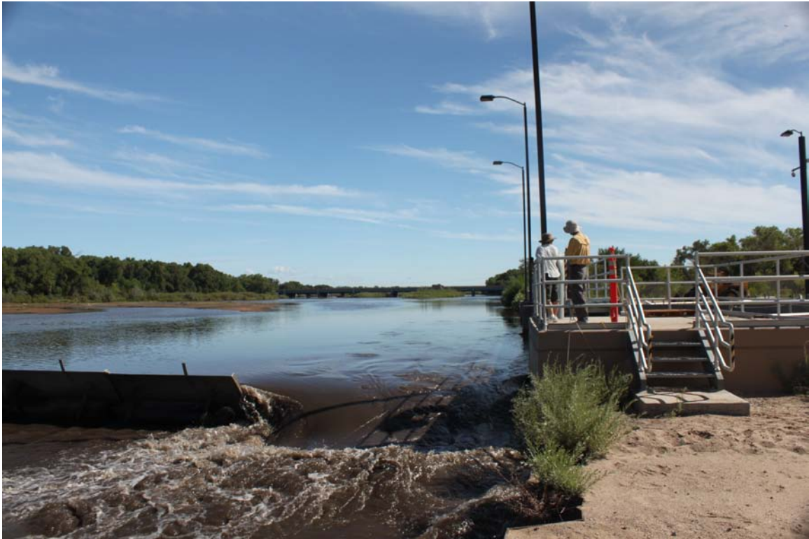
3. Looking north – close-up of water passing the drinking water diversion
