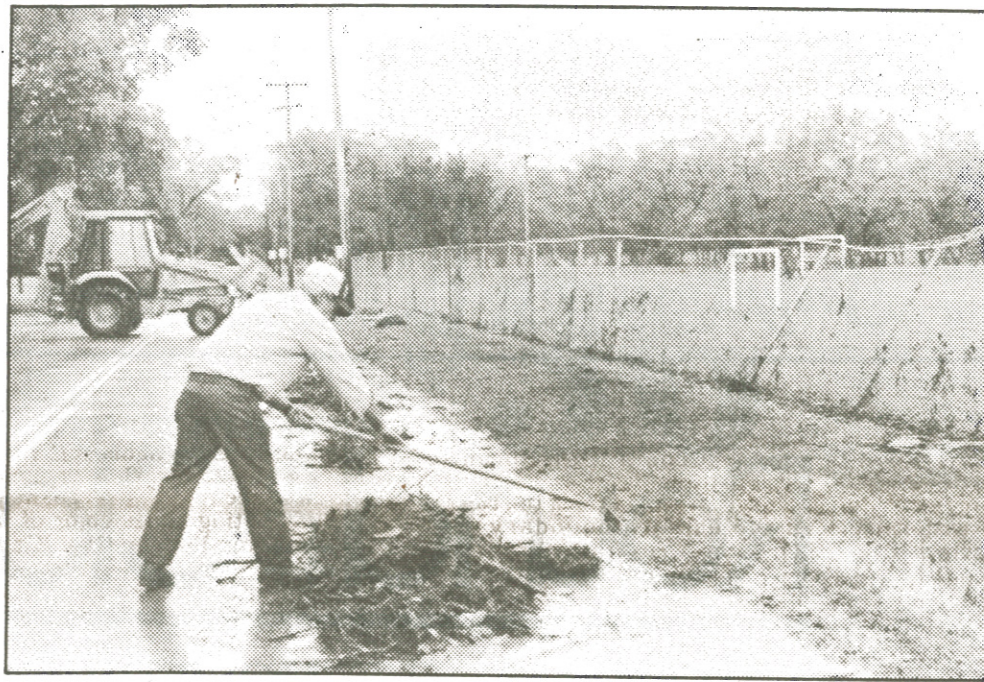
Skiatook crews clean debris trapped by the fence on the north side of Zink Park.
