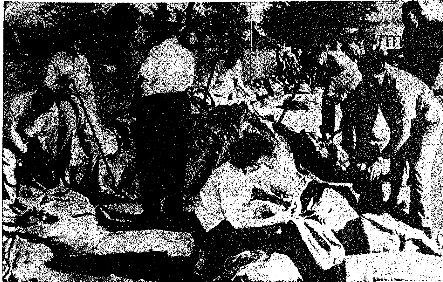
Women helped sandbag crews erect a barrier to the flooded Arkansas river along Tulsa's Riverside drive. The workers, an unexpectedly low crest and an end to days of rain were credited Sunday with sparing the city major
