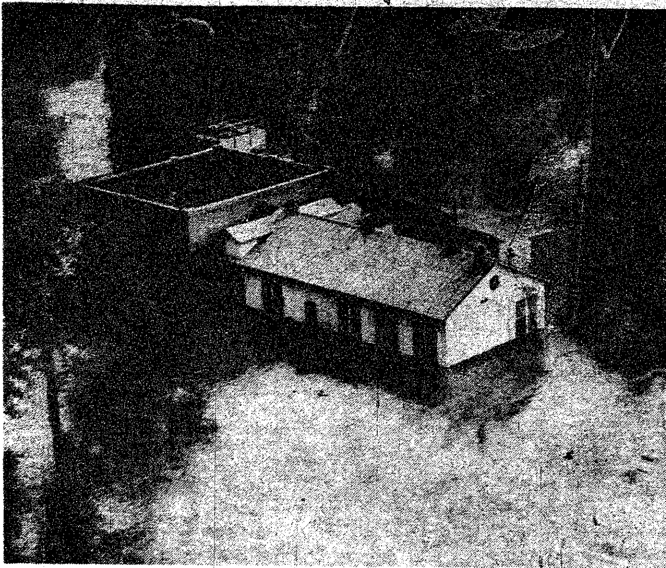
Out of Service The Anadarko power plant, above, went out of service Wednesday afternoon when Washita river flood waters crept into the building and grounded its generators. Twelve plant workers were rescued from the building by boat.
