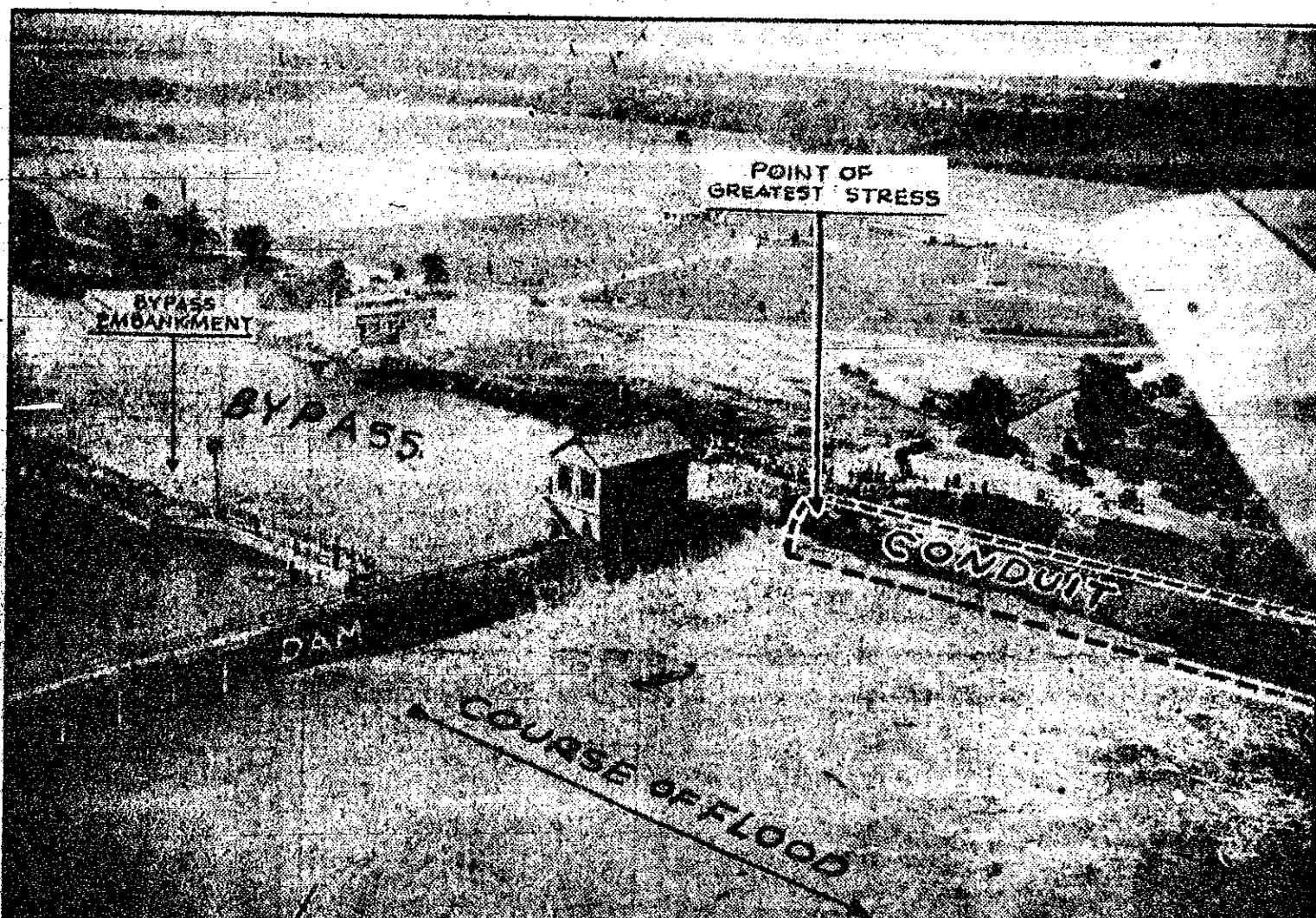
Water Cuts Around Ends of City Waterworks Dam
